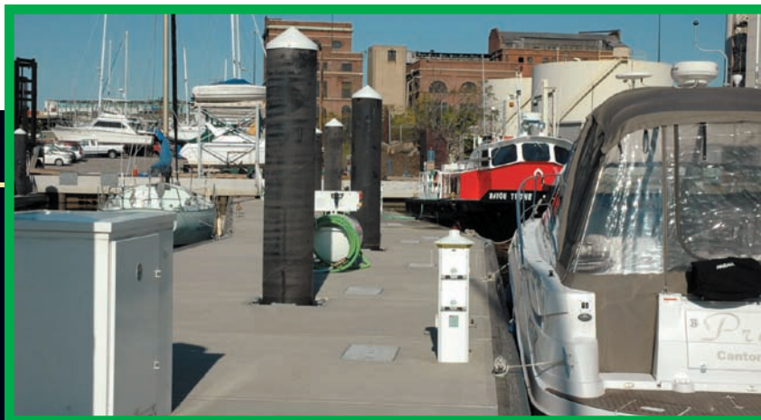
Port Covington's exceptionally large float modules will allow the marina to build a custom-designed fuel dock on this 20-ft. wide dock.
