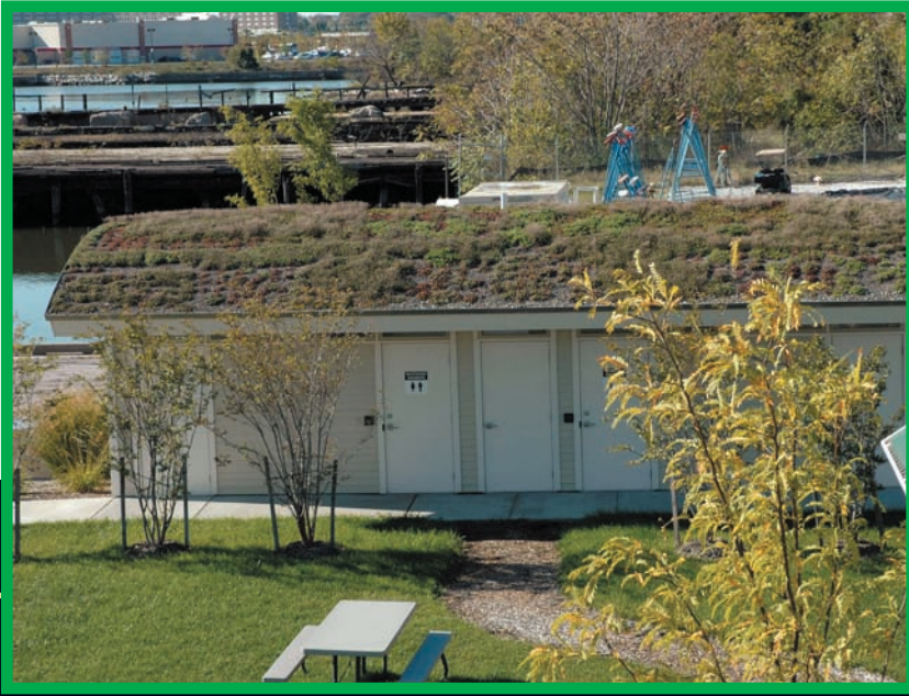
Wherever practical, Port Covington has deployed grass greenbelts and “living roofs” to capture runoff and keep pollutants out of Chesapeake Bay.
